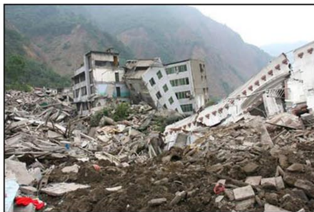
Figure 4. Total failure of concrete buildings after the earthquake hit the town of Beichuan (photo: Xinhua).
